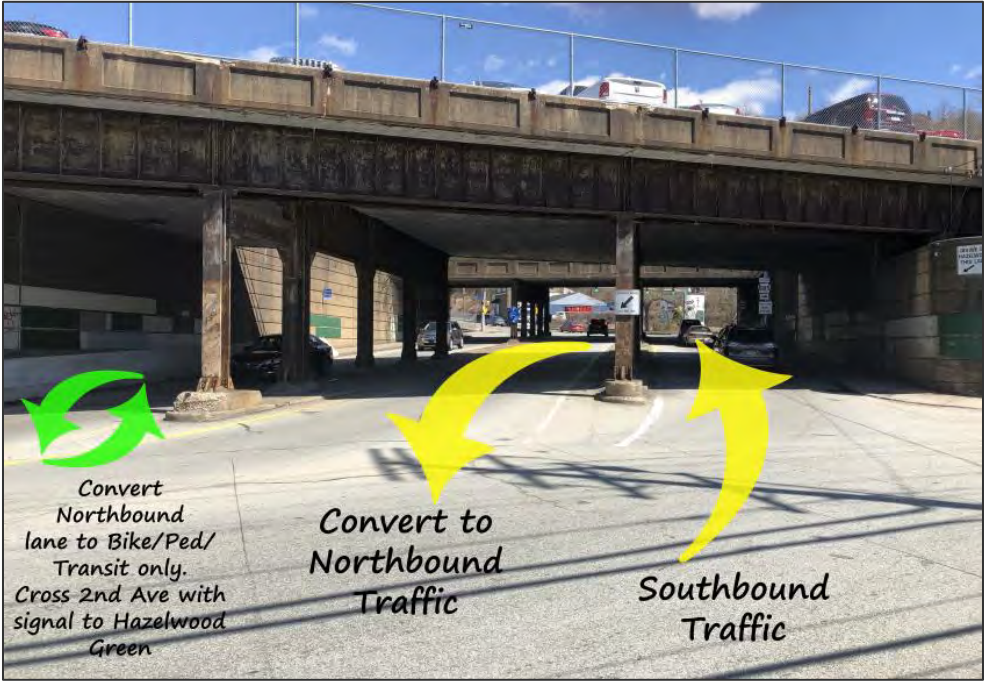
Exhibit 3-17: Bicycle/Pedestrian/Transit Lane at Irvine St/Greenfield Ave/Saline St/Second Ave (Reference Project 21 in Exhibit 3-14)
