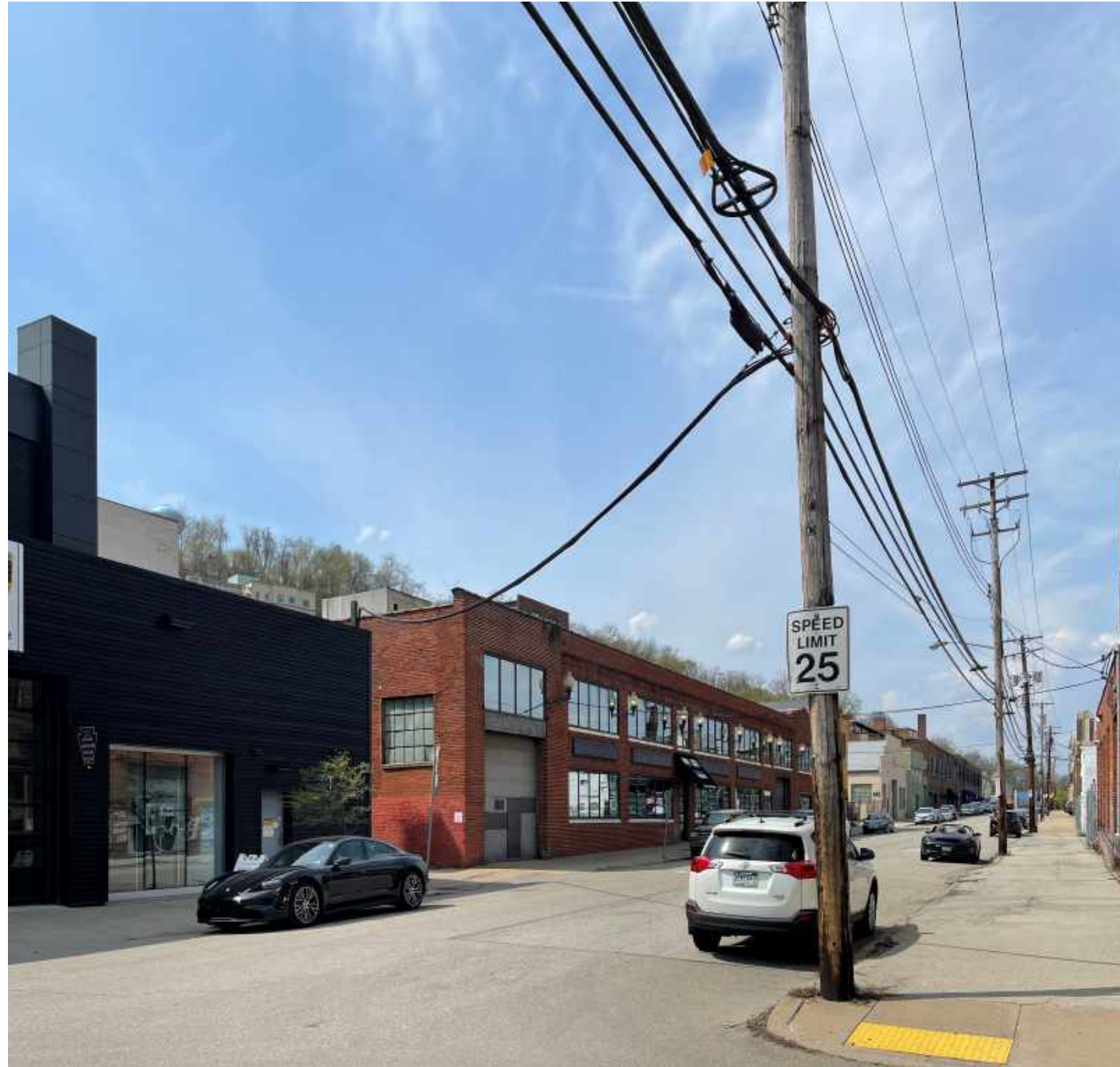
1 Street View, Existing NTS
